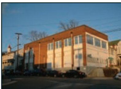
163 Main Street Action: Facade Renovation
