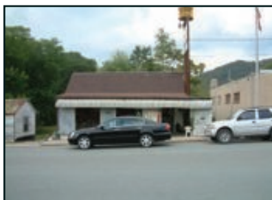
121 Main Street Action: Facade Renovation
