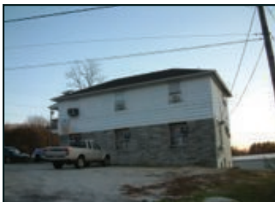
96 Main Street Action: Facade Renovation
