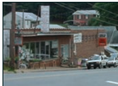
526 Front Street Action: Facade Renovation
