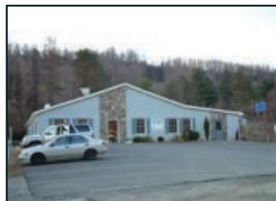
83 Tanbark Plaza Action: Facade/Street Renovation - Complete
