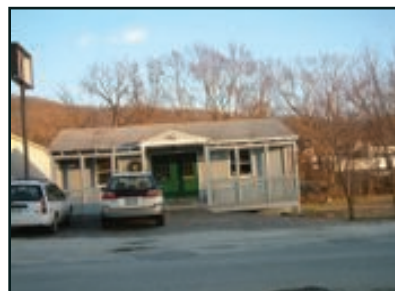
64 Tanbark Plaza Action: Facade/Street Renovation
