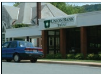
124 Main Street Action: Facade Renovation
