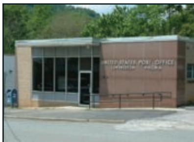
131 Main Street Action: Facade Renovation
