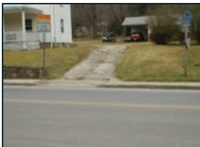
934 Front Street Issues: maintenance Action: Minor Renovation - Complete
