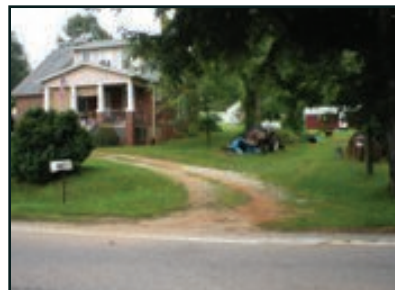
14398 James River Road Issues: outside storage Action: Minor Renovation - Complete
