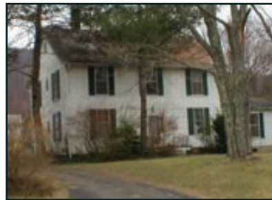
978 Front Street Issues: maintenance (painting, roof) Action: Minor Renovation
