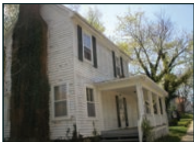
714 Front Street Issues: maintenance (soffit, paint) Action: Minor Renovation
