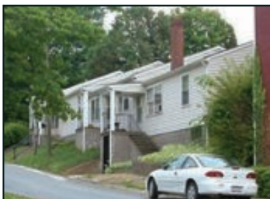
Pleasant Street Apartments Action: Facade Renovation
