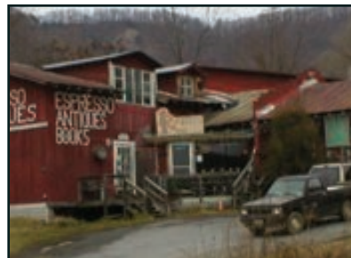
956 Front Street Issues: maintenance (railing, roof) Action: Minor Renovation
