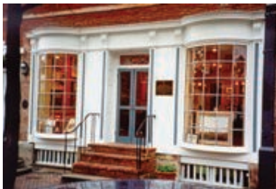
This storefront uses true materials - brick, wood cornices, and ornamental iron railings. The divided bay windows and decorative brackets under the cornice are a nice added feature.
